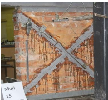
Fig. 8- Strengthening wall with GFRP
