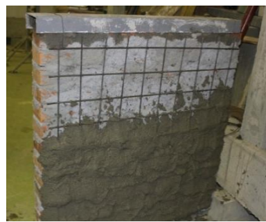
Fig. 9- Strengthening wall with layer of mortar
