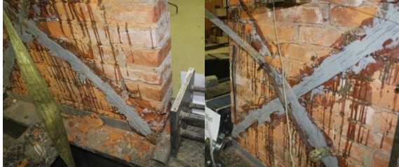
Fig.10-Failure mode and delamination of GFRP
